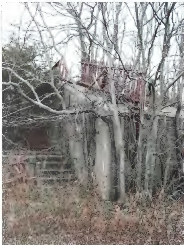
Figure 3.8. View looking northeast at gun platform #1, Battery Morris. A wood picket fence is located to the north and east of the gun platform that is painted maroon red and is in poor condition (Olmsted Center, January 2009).
